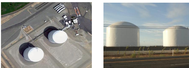
Figure 1: Suburban Propane’s two 12-million gallon double steel wall refrigerated propane tanks, separated from four 60,000 gallon pressurized tanks (LH picture, top right), by an earthen berm. Elk Grove, CA
