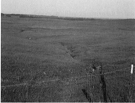
Figure 4. Typical existing channel drainage (Manning's n = 0.025 ).
