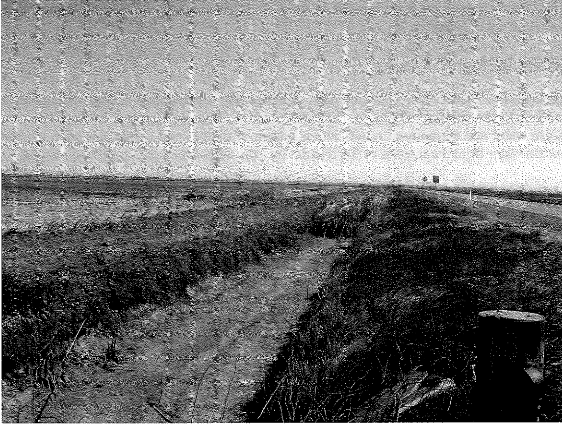
Drainage Canal along Riego Road Sutter County
