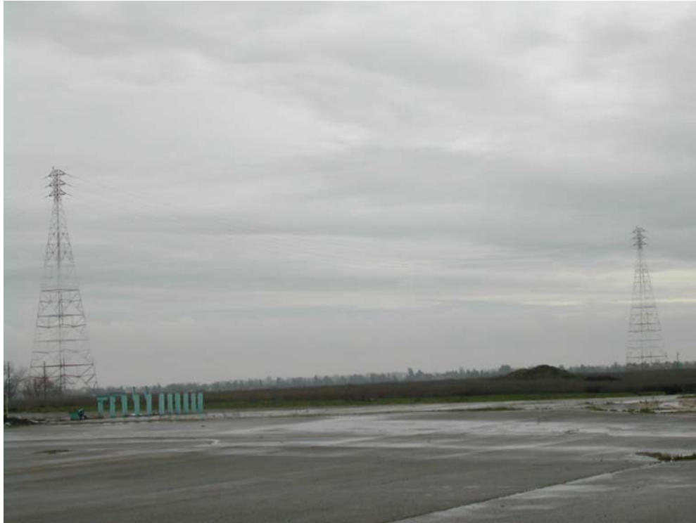
Figure 4.2.2.4 115 kV Deepwater Crossing 237' Towers on Either Sides of Channel
